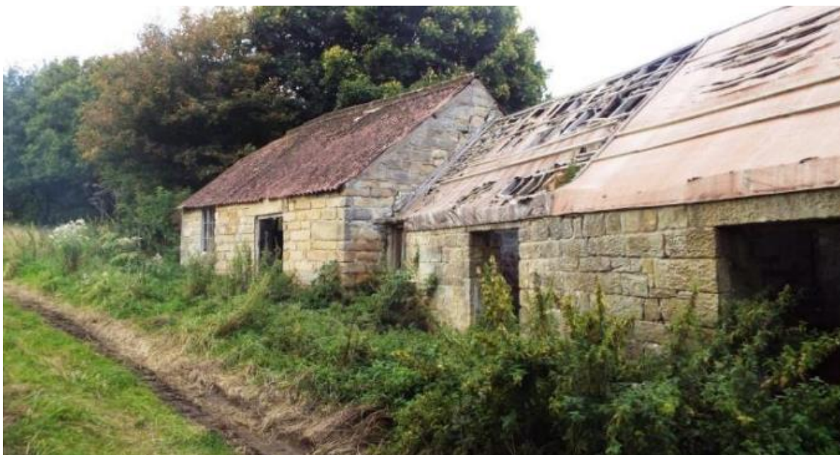
Figure 4 - Front elevation taken from the structural survey submitted for 15/01299/fl Coursed stone, tooled finish, punch faced.
